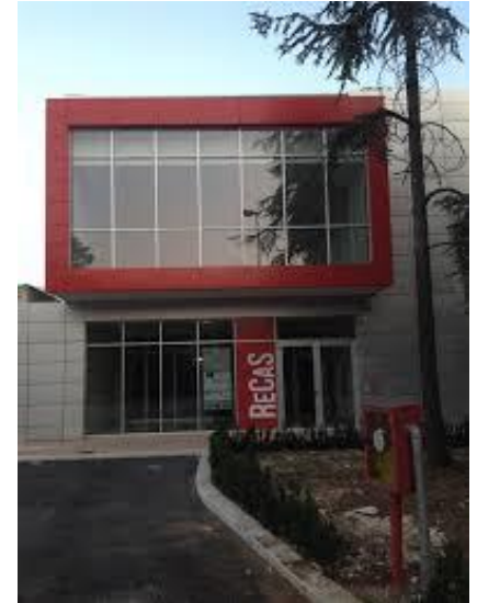
Recas DataCenter at UNIBA
