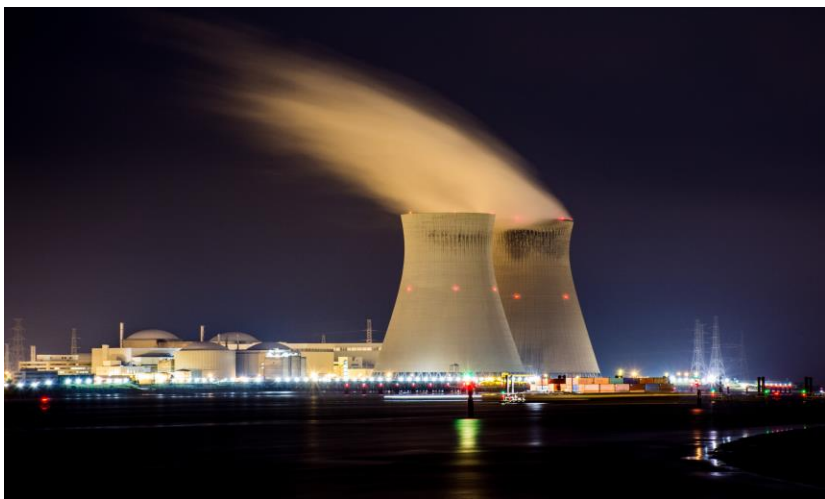
(a) Doel Power Plant, Belgium (Credits: Nicholas Therpen).
