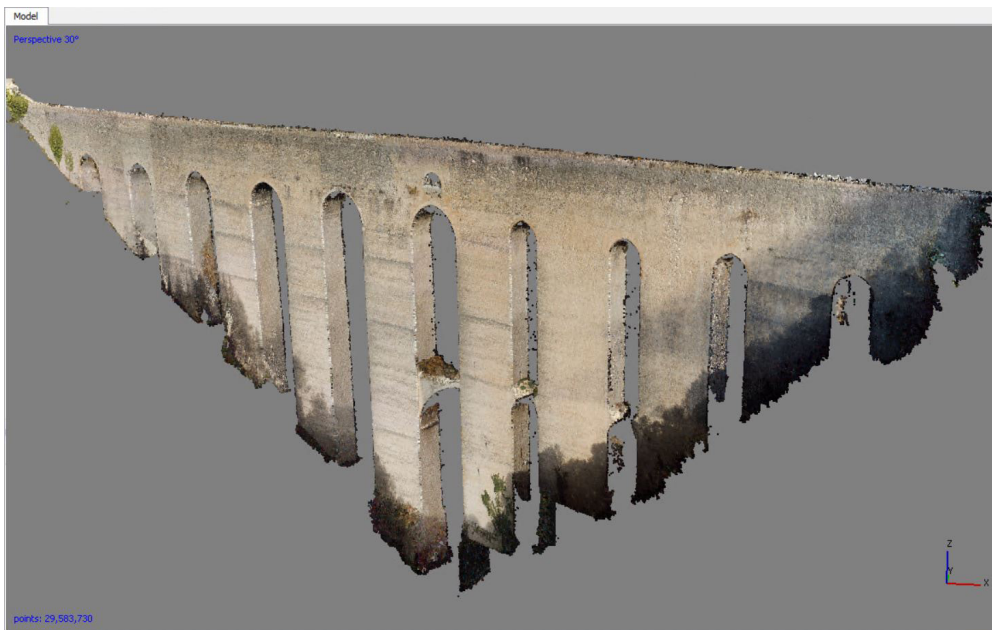
Fig. 3 Dense cloud of the South side of the Bridge of the Towers in Spoleto.
