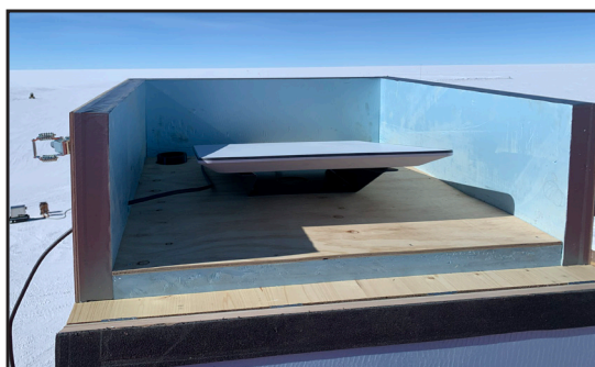
Fig. 5 Starlink antenna inside the insulation enclosure
